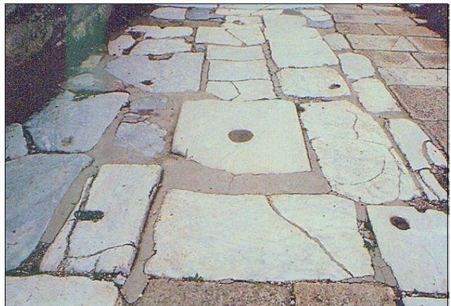
Where residents of Ephesus walked. The holes allowed the blocks to be tipped so pipes underneath could be serviced.
